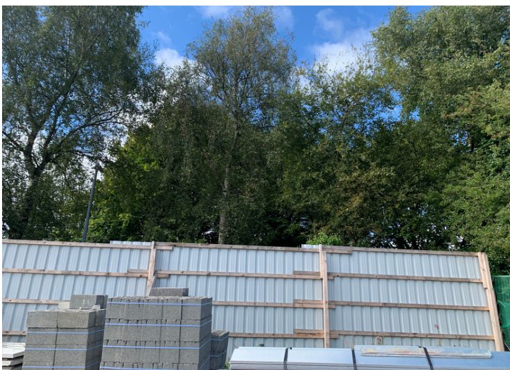
IMAGE 4: MATERIALS STORED OUTSIDE OF TREE PROTECTION FENCING
