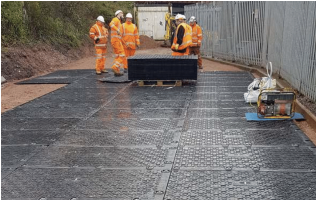
IMAGE 3: MAT GROUND PROTECTION
