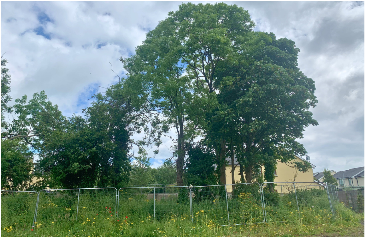
IMAGE 2: EXAMPLE TREE PROTECTION FENCING, HERRAS TYPE
