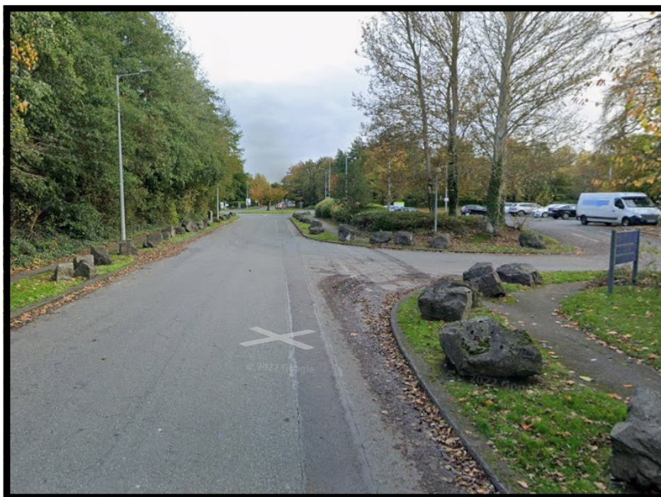
Figure 2.1 – Local Road at Site (View South to Seatown Rd) (Google)
