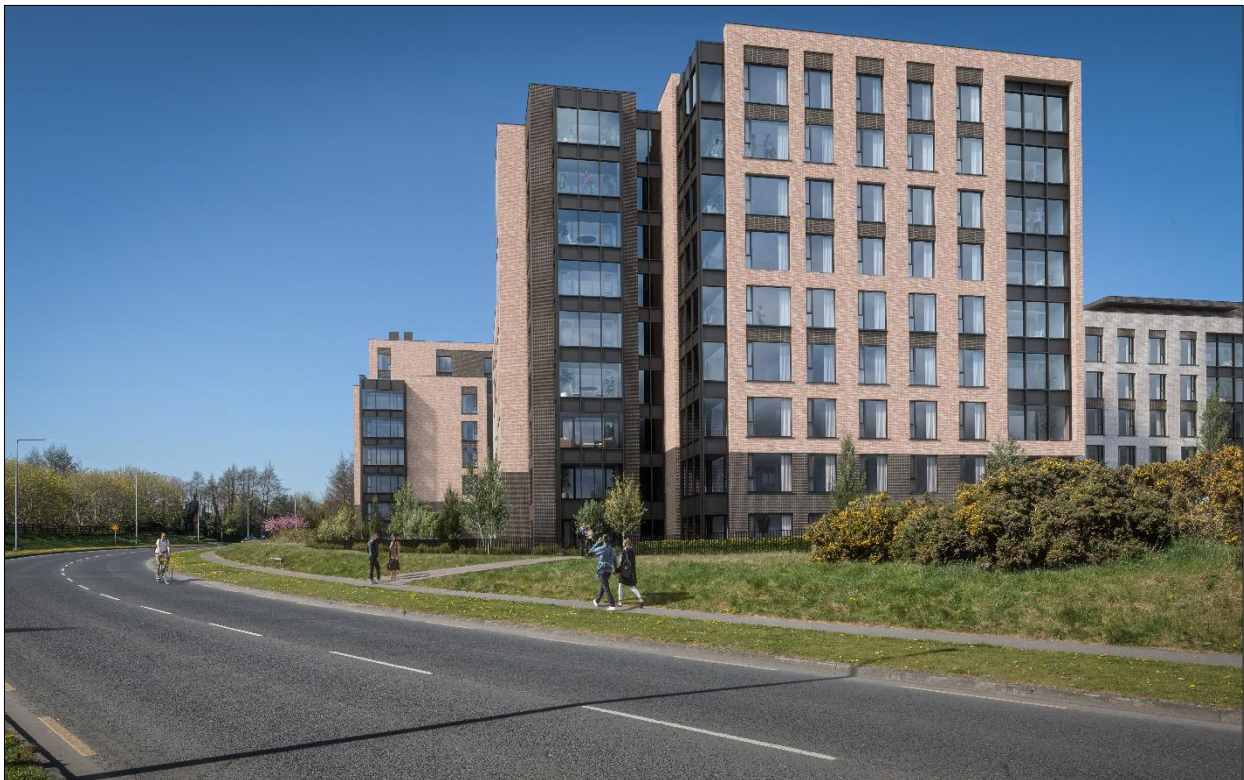
Figure 16: The façade treatment of Block D when entering the Swords urban area from the east
