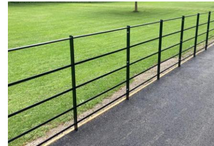
Boundary Type 2 1.2 m High Estate Metal Railing Fence
