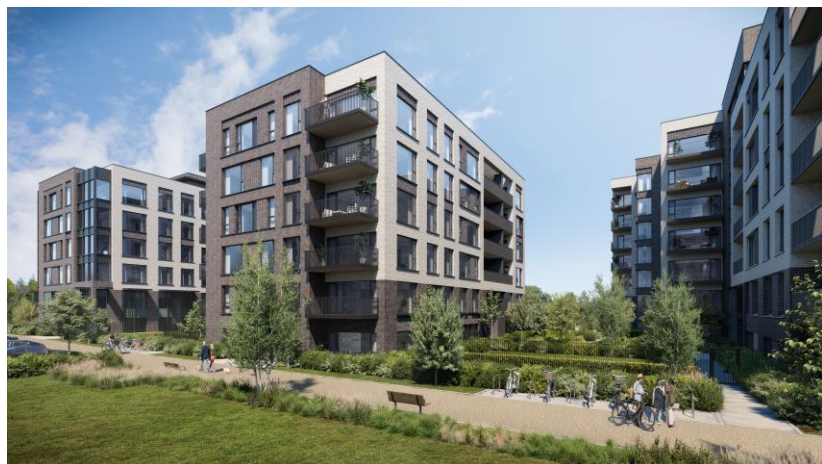
Indicative image looking to the central area of the Site - Blocks A-C (source: 3D Design Bureau)
