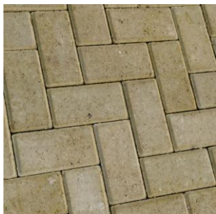
Permeable Block Paving / Parking Bays
