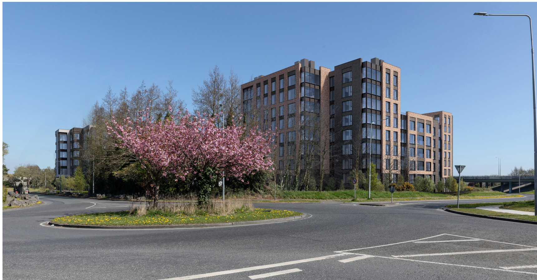
Figure 52. CGI showing the southwestern corner of the development viewed as approached from Swords town centre along Mantua Road. Source: 3DDB 2026.
