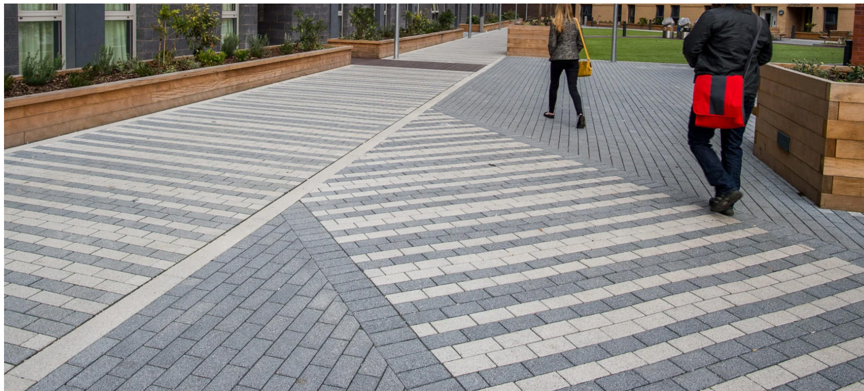
INDICATIVE: PERMEABLE PAVING TO HARD LANDSCAPED AREAS
