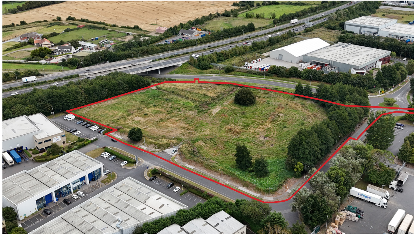
Figure 11. Aerial Photo from North West; M1 Motorway in background
