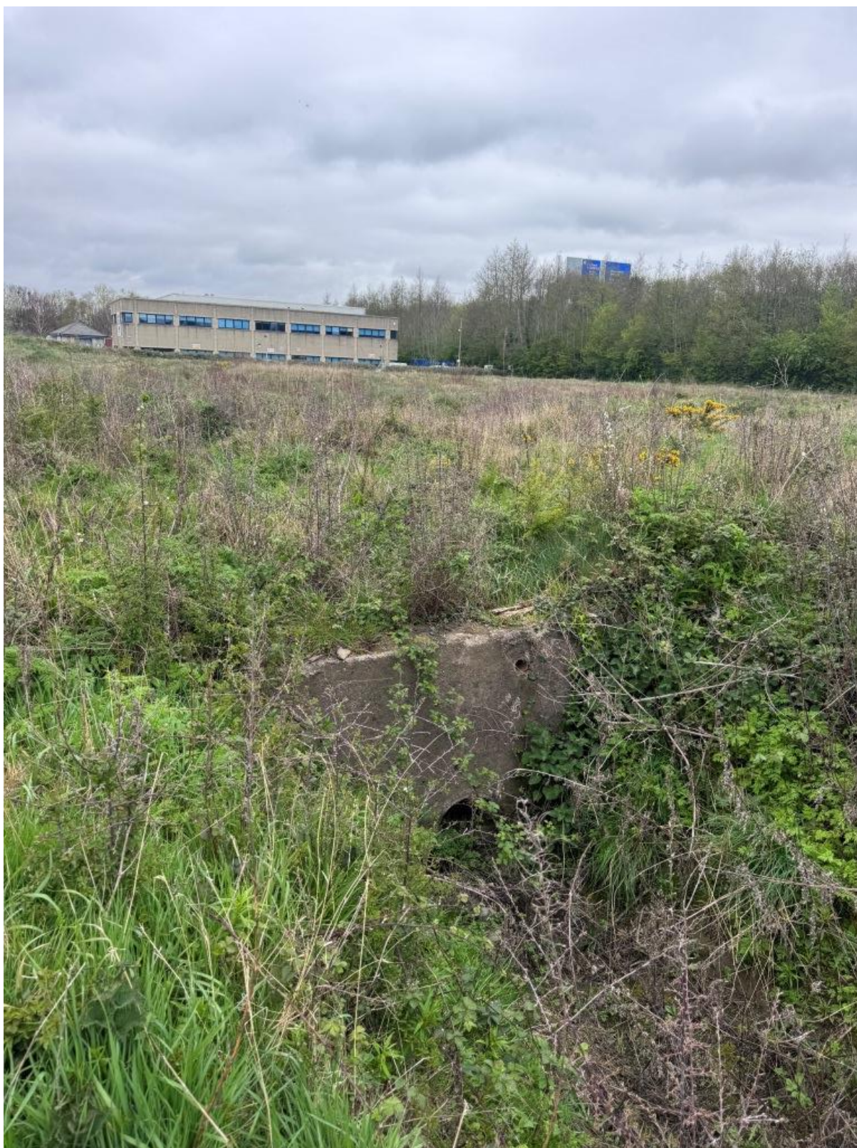
Plate 4: Drainage culvert within the central and south-east portion of the development site.
