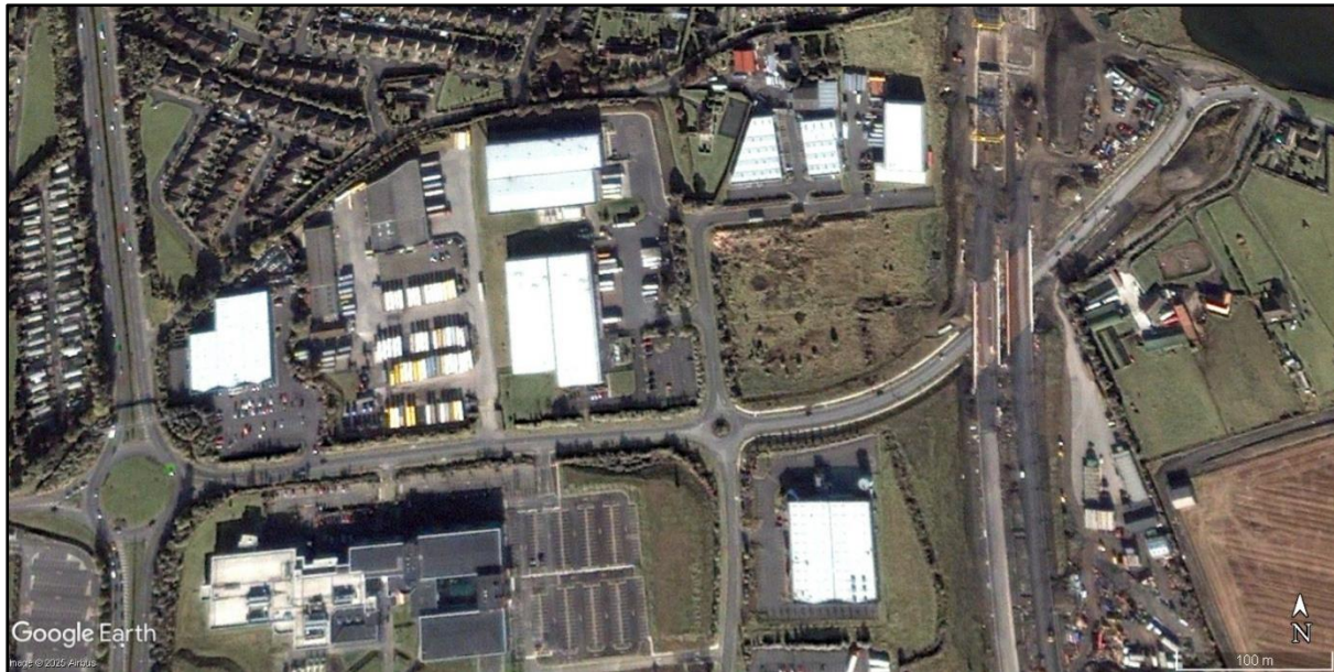
Figure 9: Aerial image centred on proposed development area from October 2002 with ongoing construction of the M1 motorway visible to west of subject site. (Source: Google Earth Pro)
